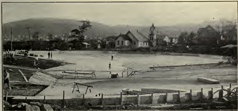
THE JOHNSTOWN POOL, UNDER CONSTRUCTION
